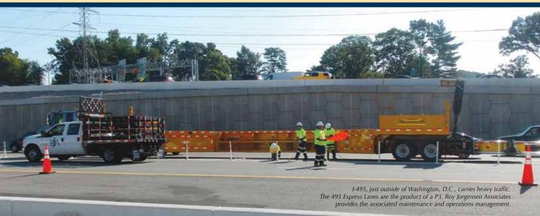
is done. The barrier's 5-foot-high walls prevent drivers—even those in high-profile vehicles—from seeing into the work zone. These benefits not only help prevent work-zone traffic incidents, but also reduce complaints from passing motorists because the work zone is less disruptive to their travel.
