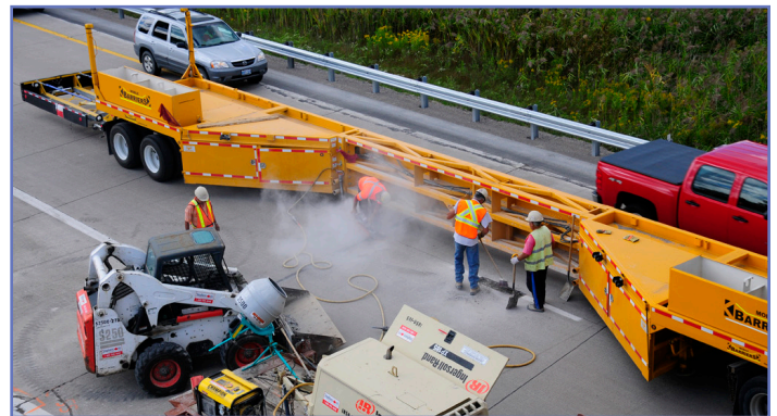
A mobile work zone barrier being moved into place for Highway 115 road work.
