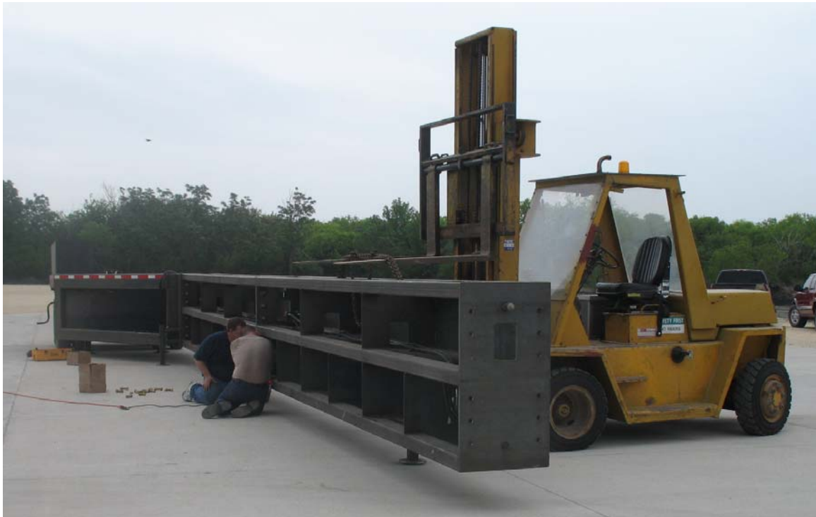
Figure 2.4 – Assembly Process of Wall Panels
